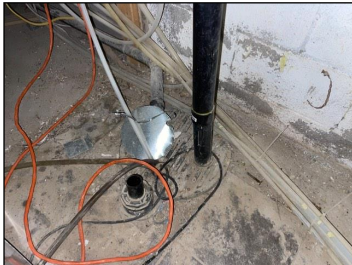
34. Solid waste pump (ejector pump)
