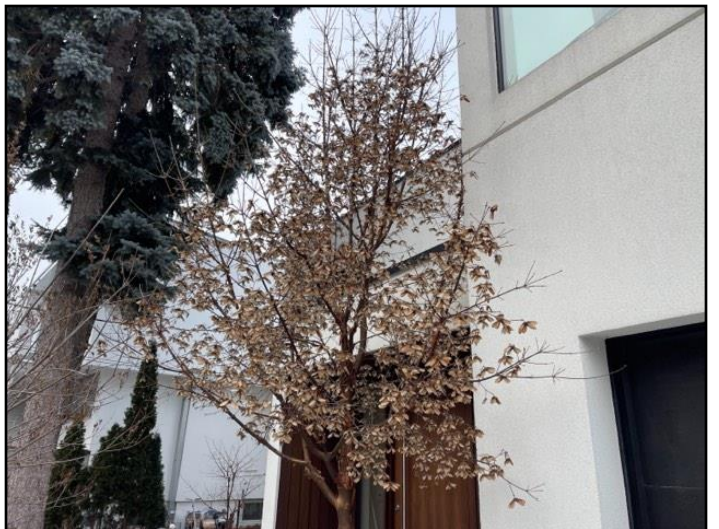
6. Trees or shrubs too close to building
