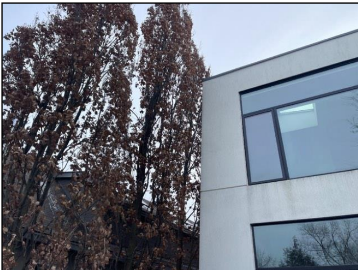
5. Trees or shrubs too close to building
